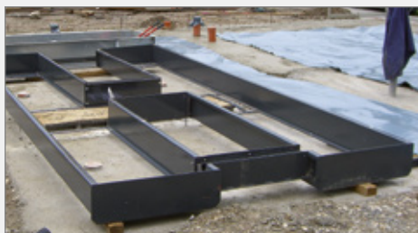
Mounting frame for runway versions with or without floor compensation for accurate lift fitting. The prefabricated channel-section frame gives high precision during installation.
